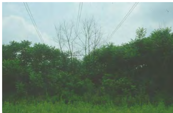
Figure 7. Trees and people should not reach the electric conductors.
