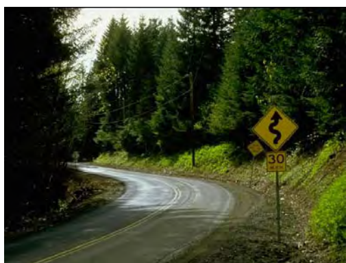
Figure 6. Vegetation management improves appearance and road delineation.
