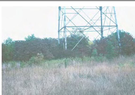
Figure 8. Structure inspection and maintenance is made easier with vegetation control.
