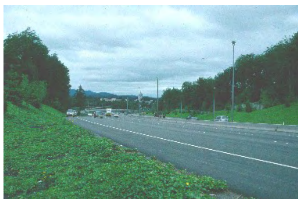
Figure 1. The safety recovery zone is an integral part of the highway design.
