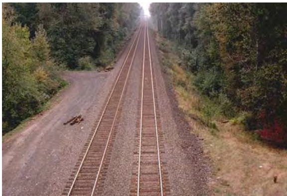
Figure 12. Vegetation control in roadway ballast preserves ties and track stability.
