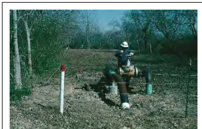
Figure 15. Vegetation control enables pipeline inspection and maintenance.
