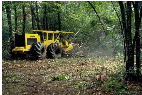
Figure 5. Some mechanical equipment can remove large trees on the right-of-way.
