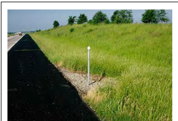
Figure 3. Total vegetation control around delineator posts facilitates mowing.
