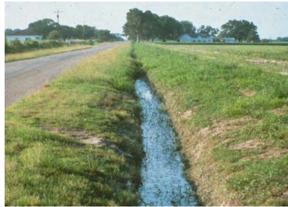
Figure 10. Grasses are encouraged in some ditches to reduce soil erosion.
