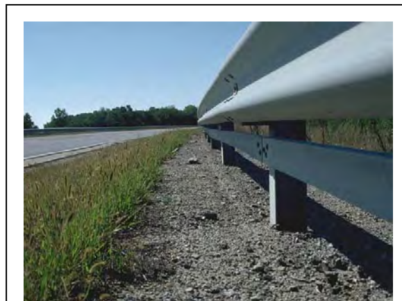
Figure 1. Guide rails need to be seen by motorists as well as maintenance
